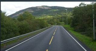
Roadways and other paved surfaces
